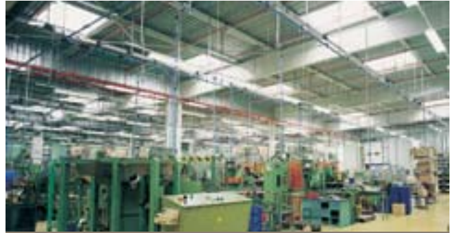
Assembly workshop Transair Ø 63 and Ø 25
