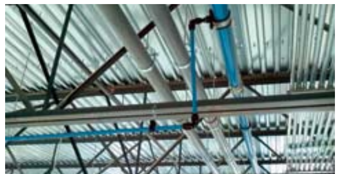
Alternative energy Transair Ø 76 and Ø 63
